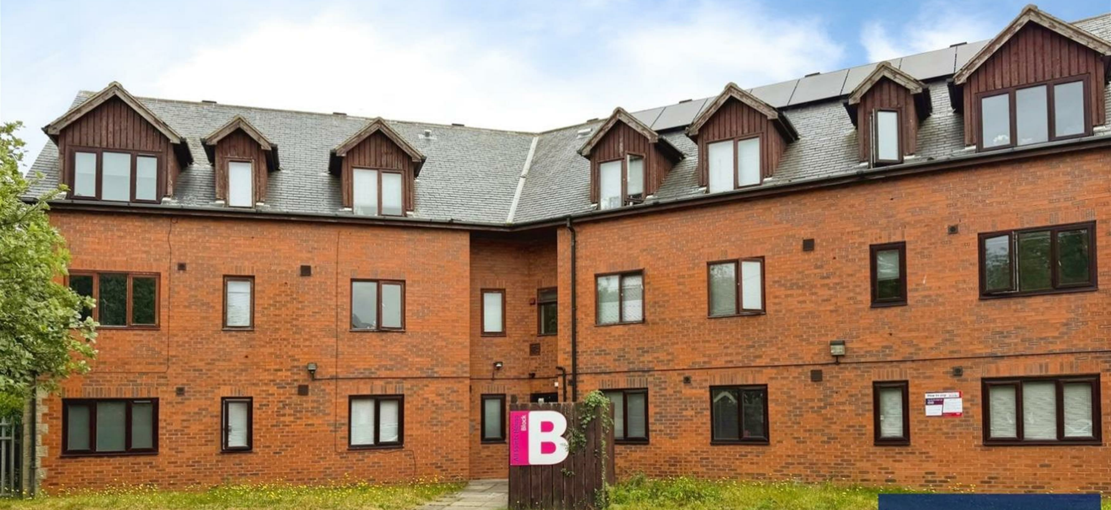
All Saints House Block B, Portobello Lane, Sunderland, SR6
